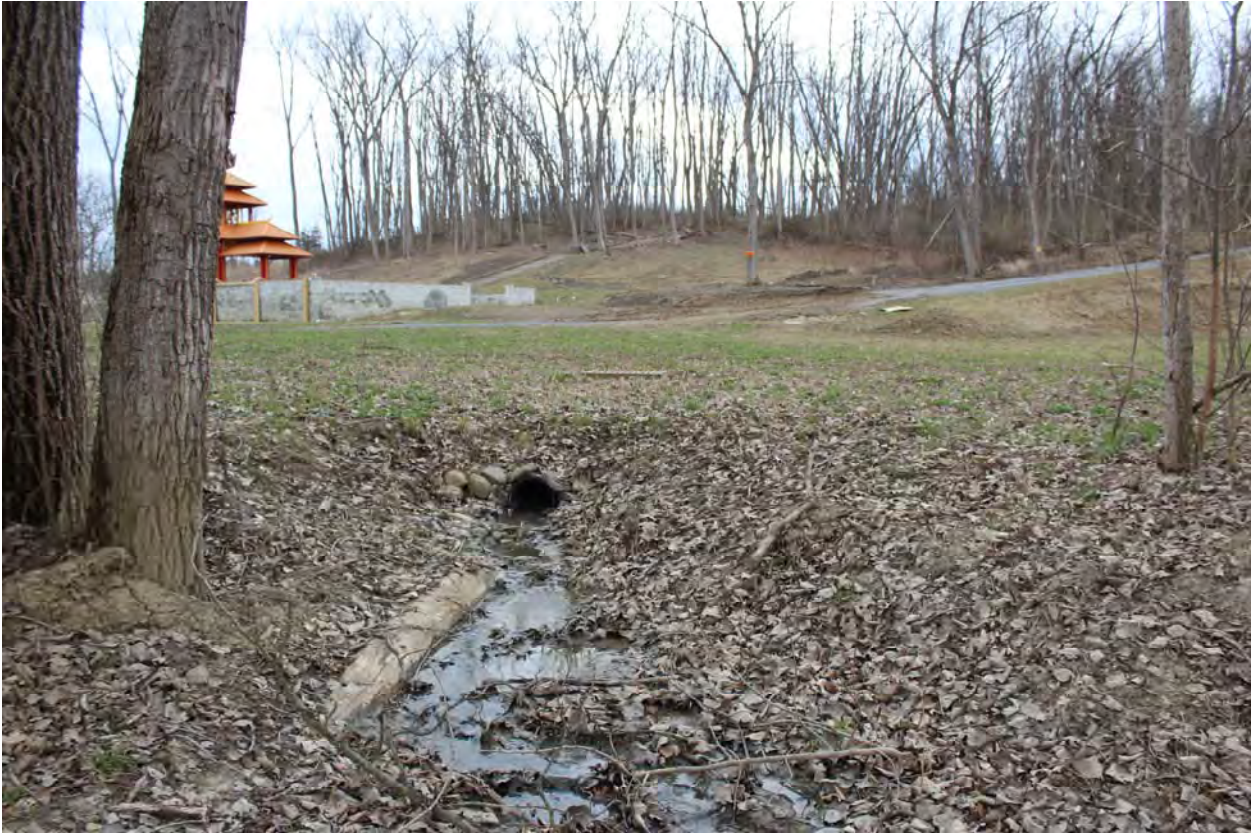
Photo 12. View of stormwater drain in Area 1, facing southeast.
