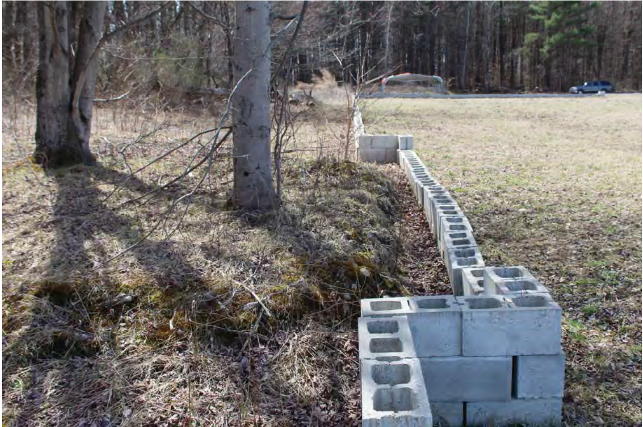
Photo 29. View along the eastern concrete block wall at Area 3, facing south.
