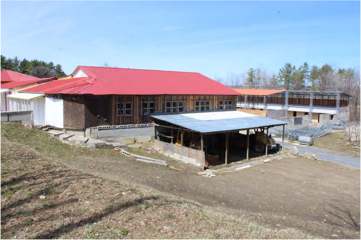
Photo 48. View of slope descending from the eastern part of Area 4C, facing northwest.
