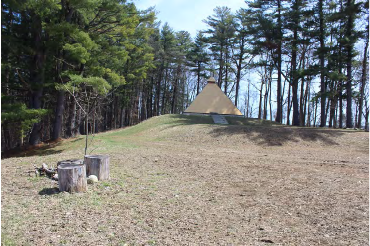
Photo 49. View of the existing water storage pyramid showing terraces, facing southeast.
