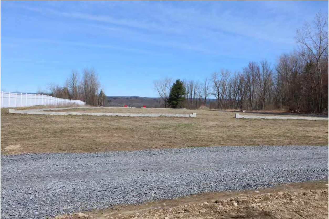
Photo 64. View of where the proposed water line from Area 4A will connect with Area 3, facing north.
