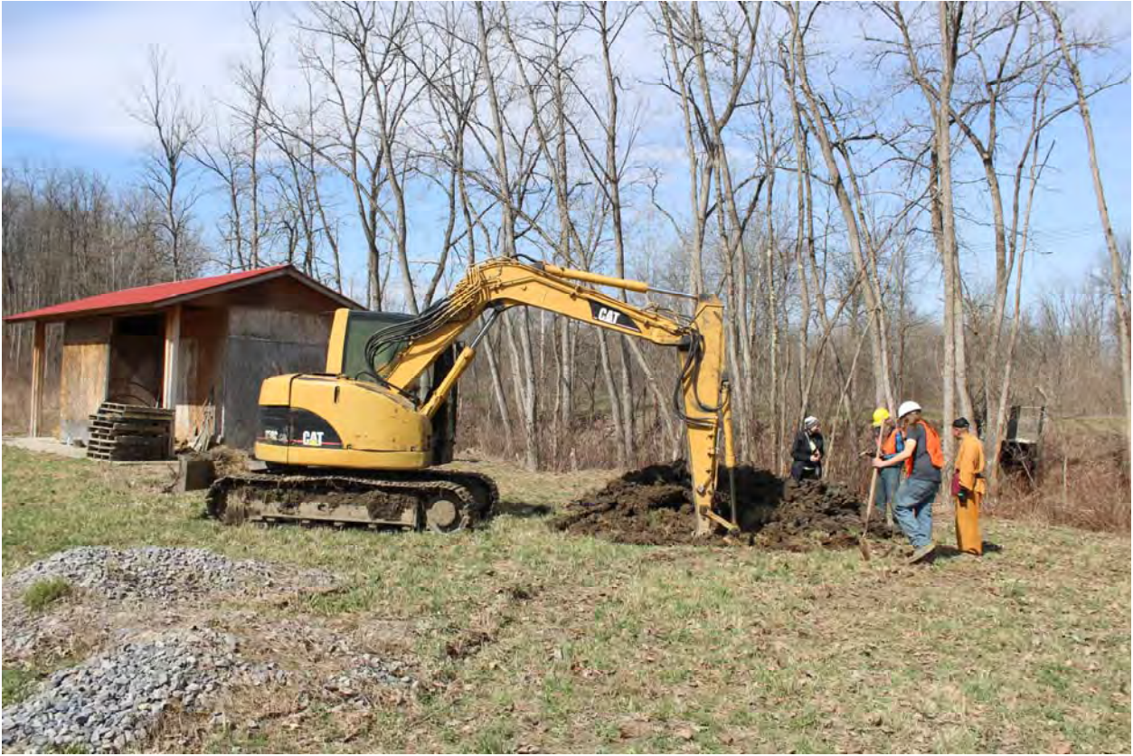
Photo 1. View of the excavation of Trench 1 at Area 1, facing southwest.
