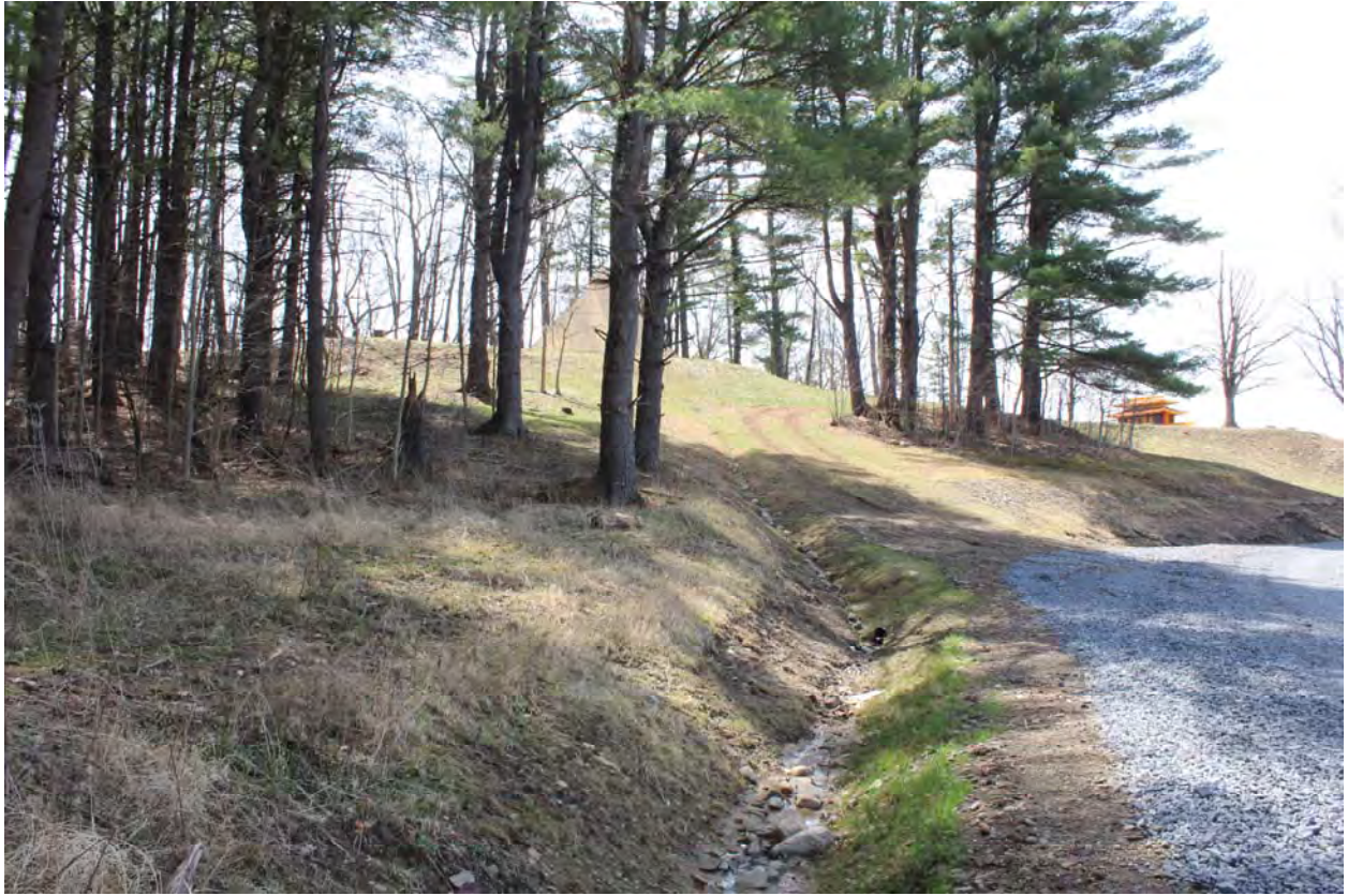
Photo 51. View from the north end of the T Transect at Area 4C, facing south.
