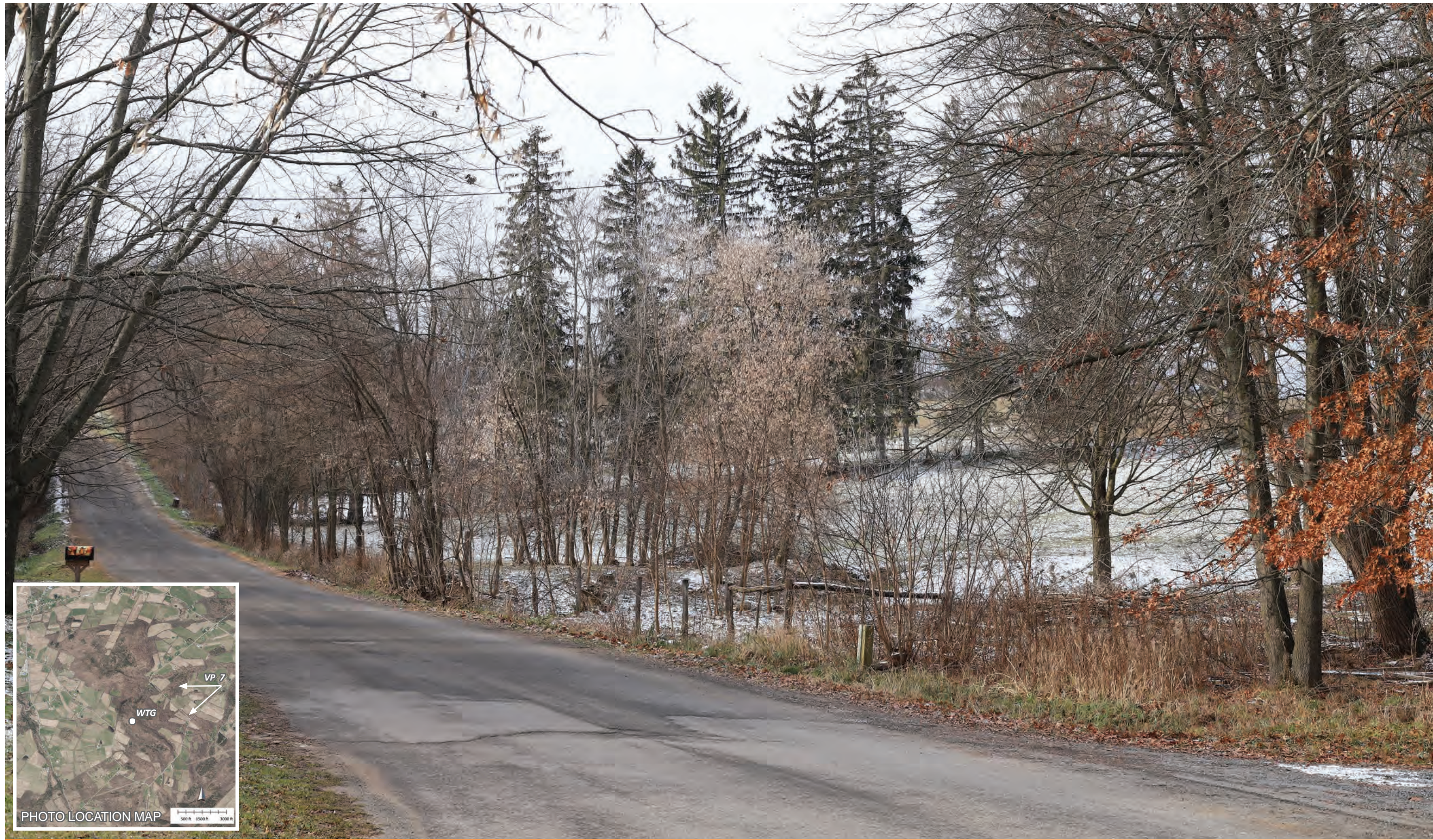
VP 7- ROUND BARN ROAD EXISTING CONDITION
