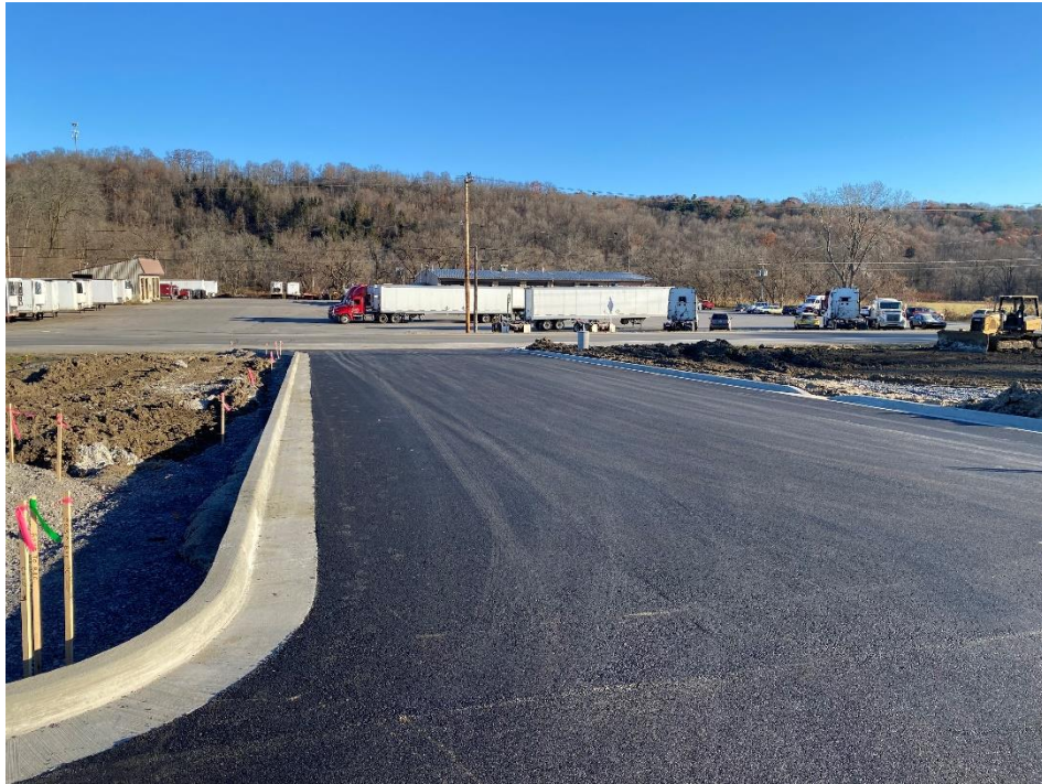
Figure 7 - View of western driveway, looking north.
