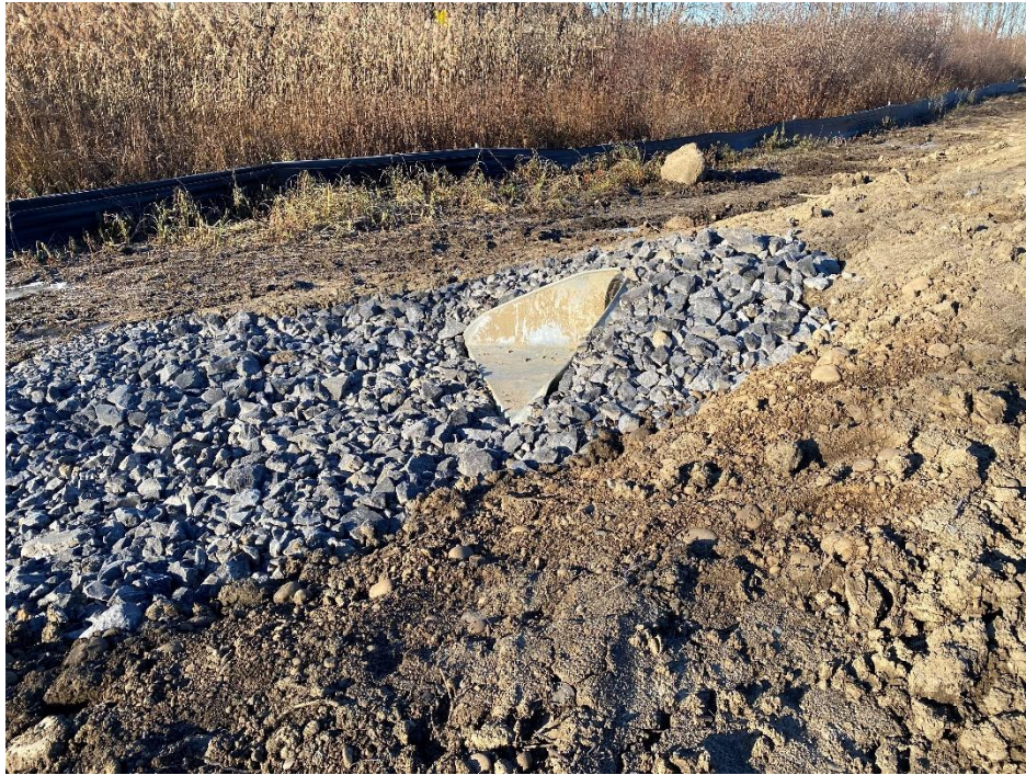
Figure 5 - Outlet for southern stormwater pond.
