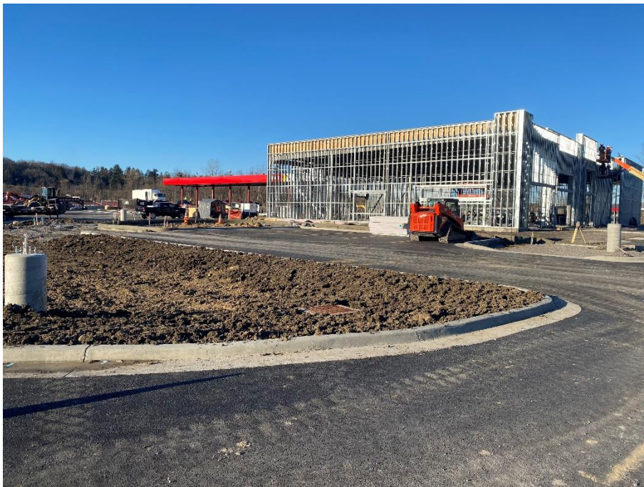
Figure 2 – View of building and drive thru area, looking southwest.
