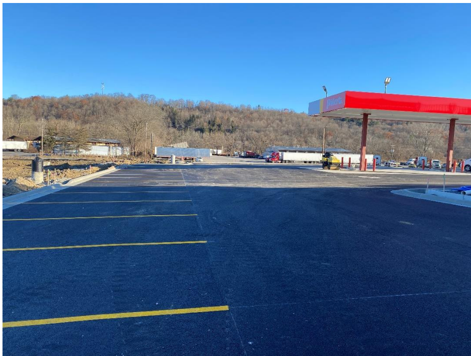
Figure 6 - View of western half of front parking lot, looking north.
