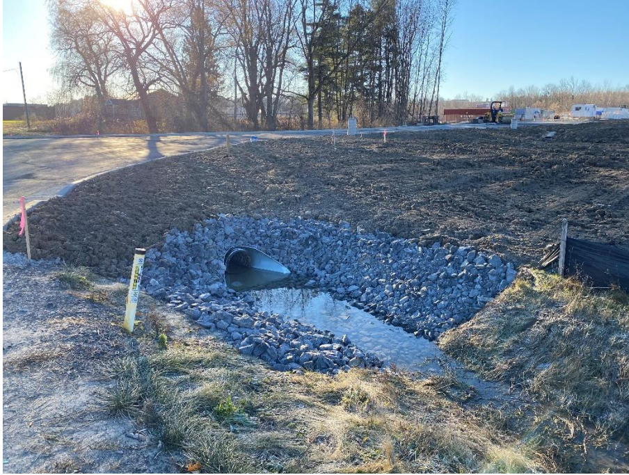
Figure 1 – View of culvert beneath the eastern driveway, looking southeast.
