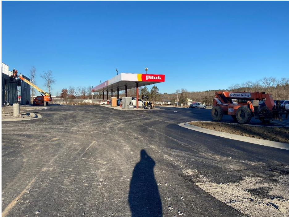
Figure 3 – View of gas pump area and front parking lot, looking west.
