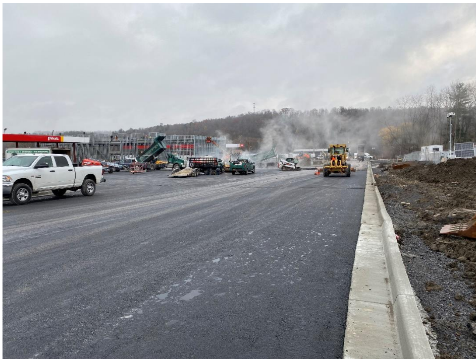
Figure 6 – View of paving work for truck fuel pump area, looking north.
