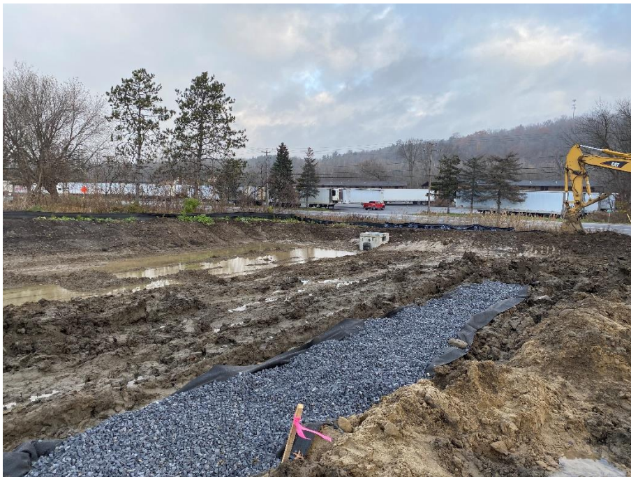
Figure 2 - View of NW stormwater pond and outlet structure, looking northwest.
