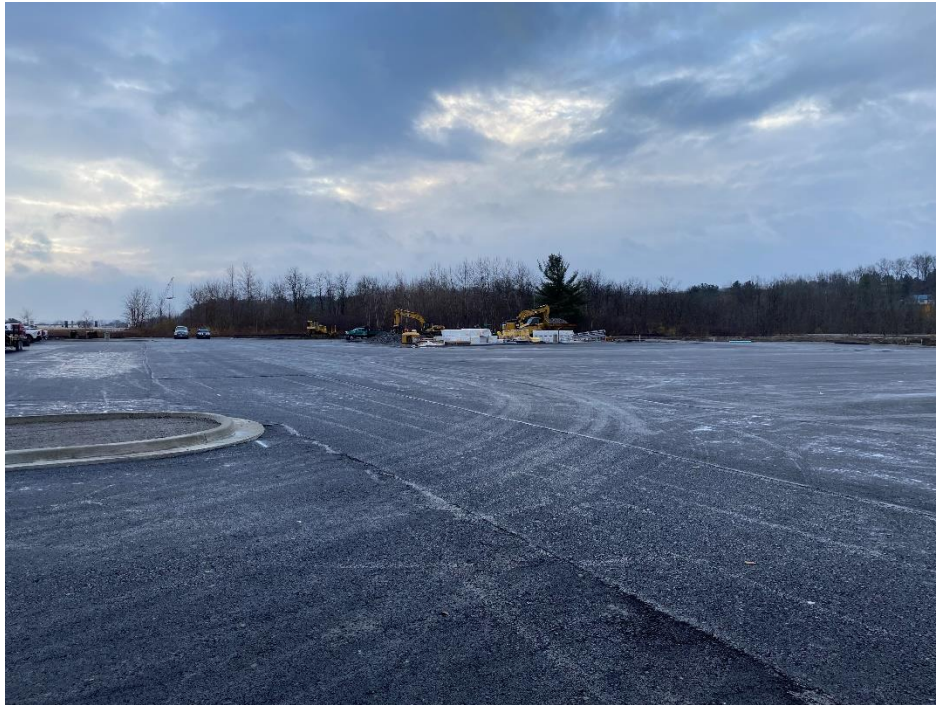
Figure 5 – View of paving for back parking area, looking east.
