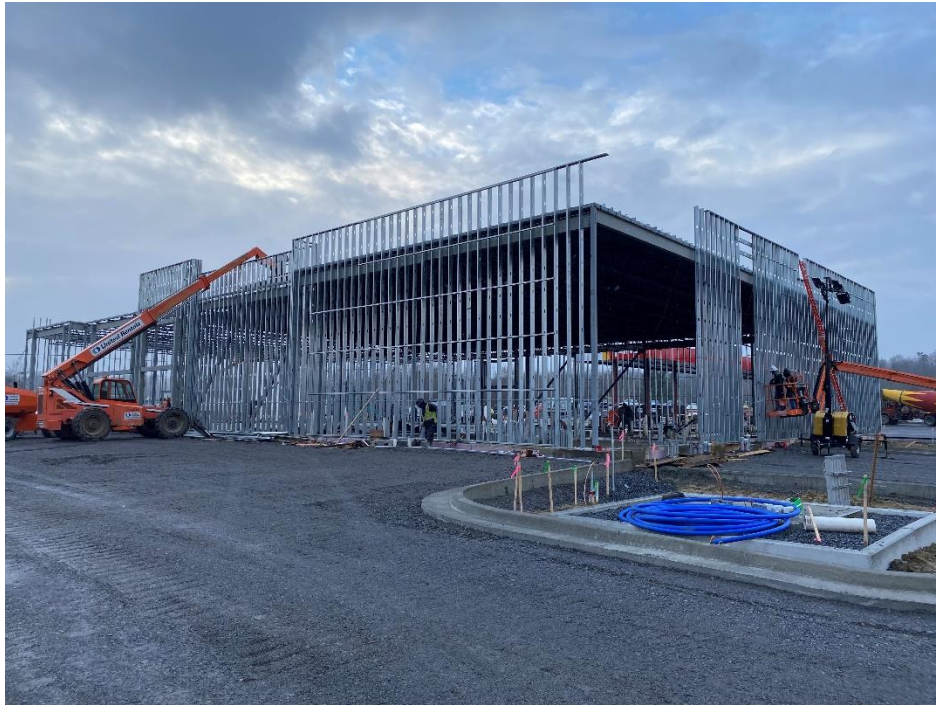
Figure 3 – View of steel erection for the main building, looking southeast.
