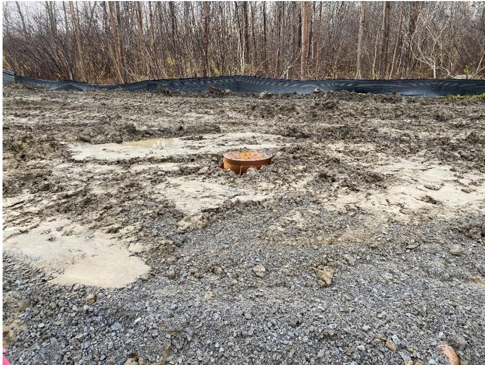
Figure 6 - Low sanitary structure raised and cover installed.
