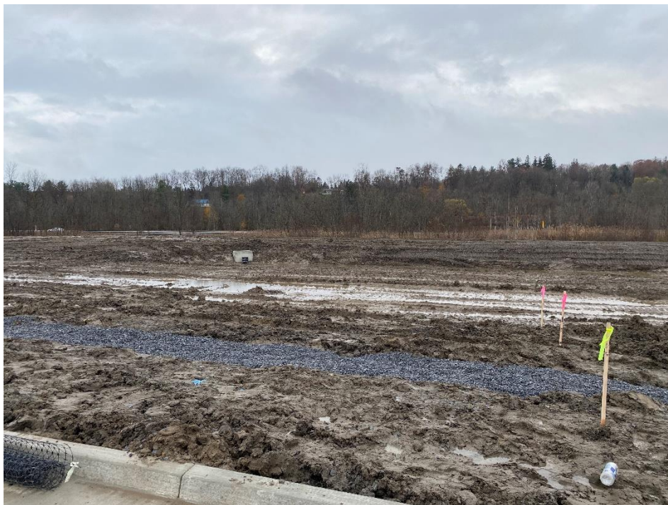
Figure 4 – View of grading and outlet structure for southern stormwater pond, looking southeast.
