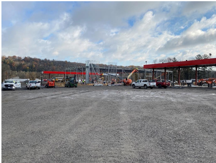
Figure 2 – View of steel erection for building, looking northeast.
