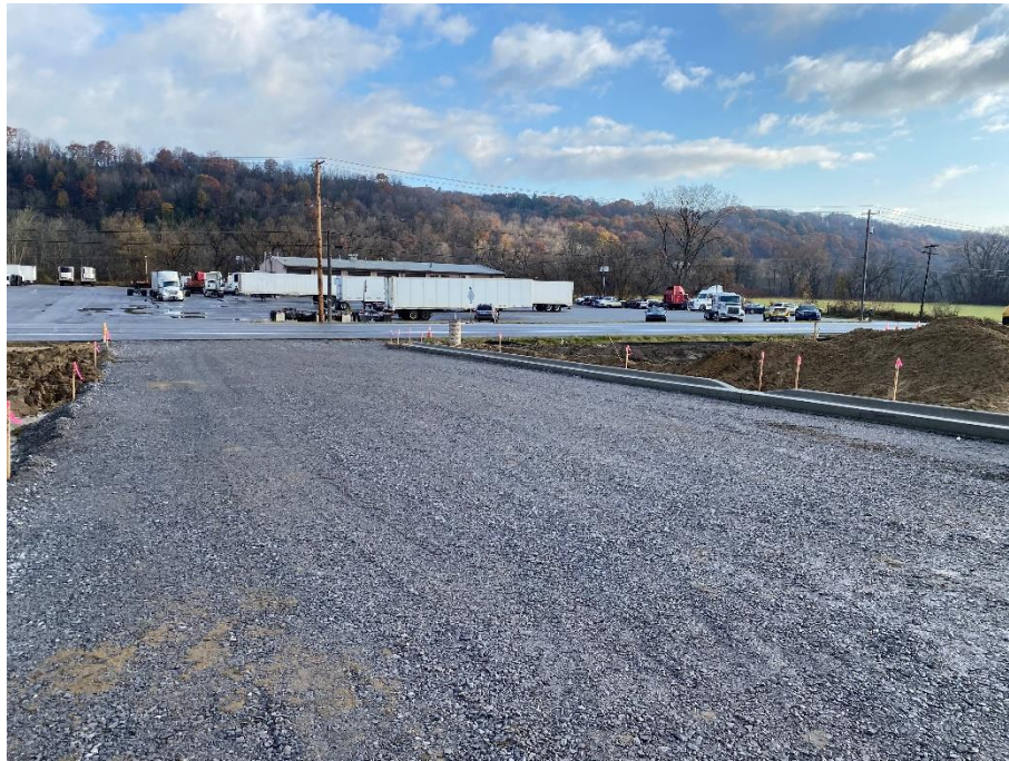
Figure 1 – View of subbase grading and new curb for western driveway, looking northeast.
