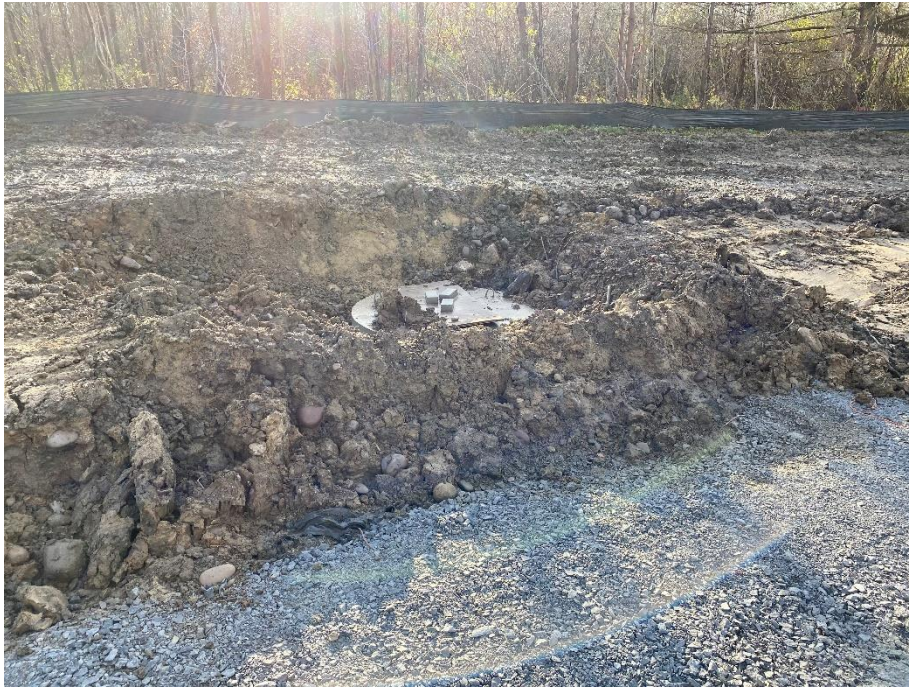
Figure 1 - Add inlet protection around low structures.
