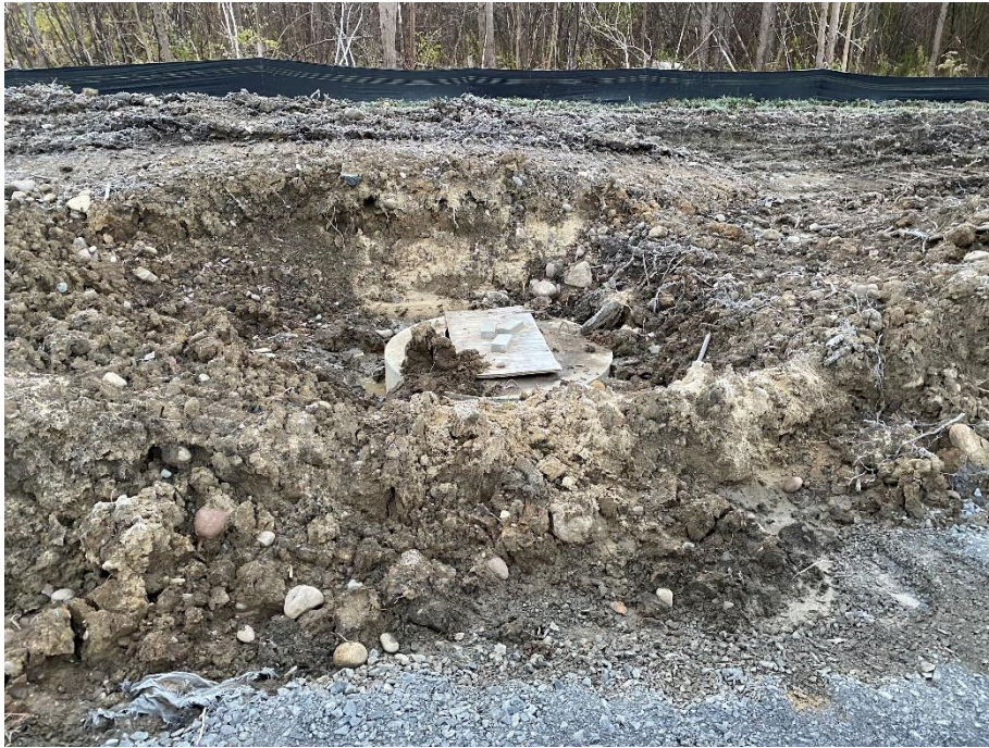
Figure 1 - Add inlet protection around low structures.
