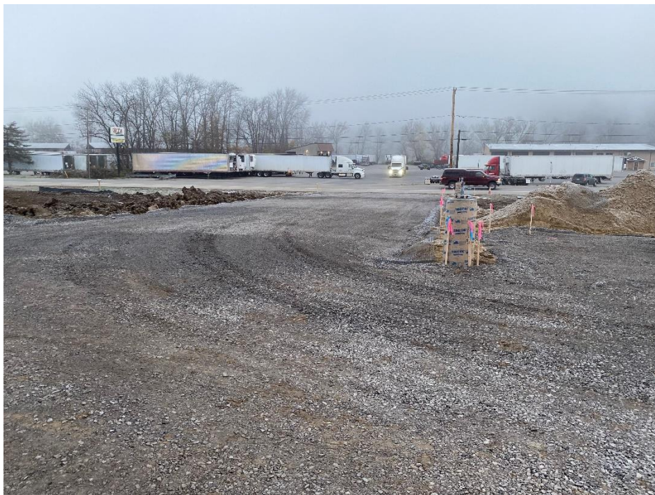
Figure 4 – View of subbase grading for western driveway, looking north.
