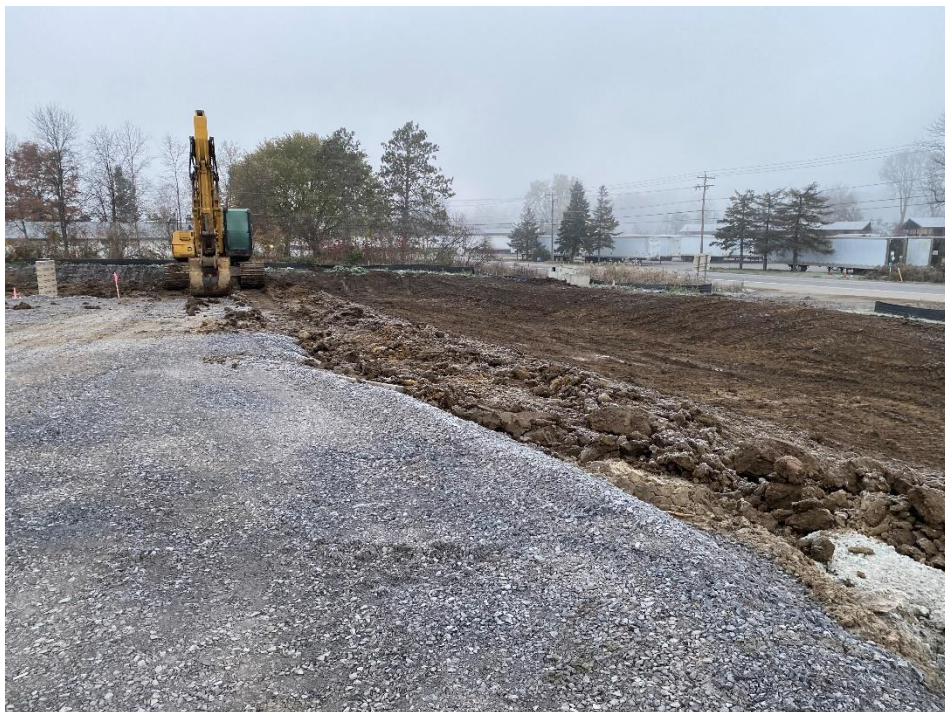
Figure 6 – View of grading for stormwater pond in NW corner of site, looking west.
