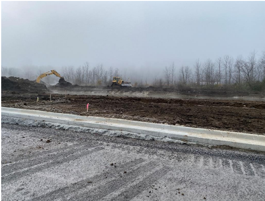
Figure 1 – View of grading for south stormwater pond, looking south.
