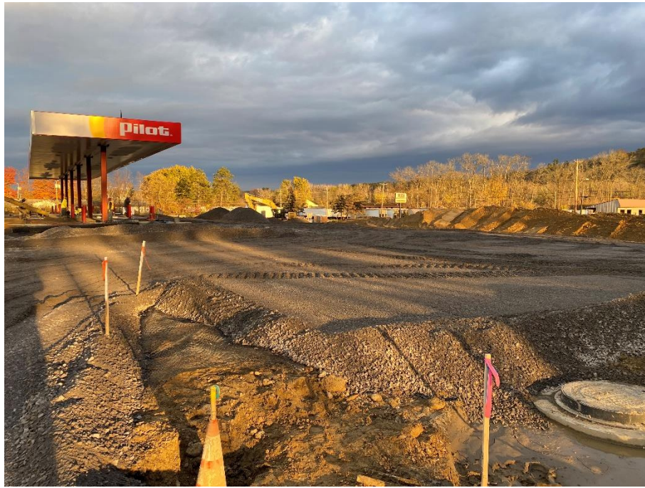
Figure 1 – View of subbase grading for front parking area, looking northwest.
