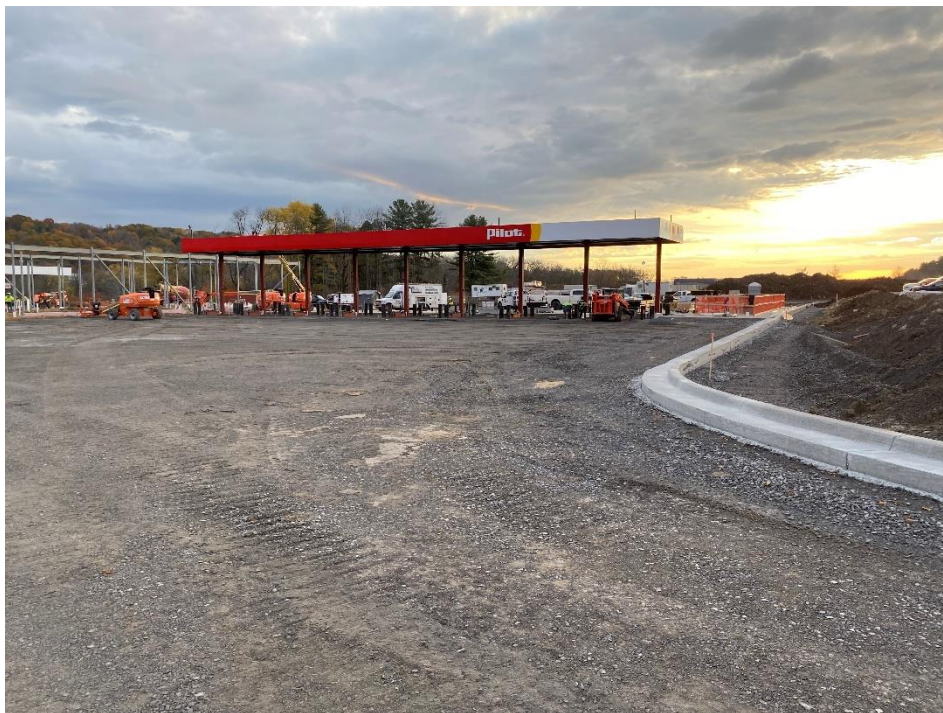
Figure 4 - View of subbase grading for truck fuel pump area, looking northeast.
