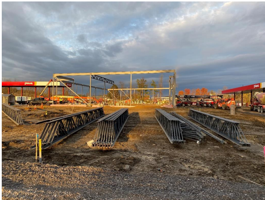
Figure 2 – View of steel erection for building, looking west.
