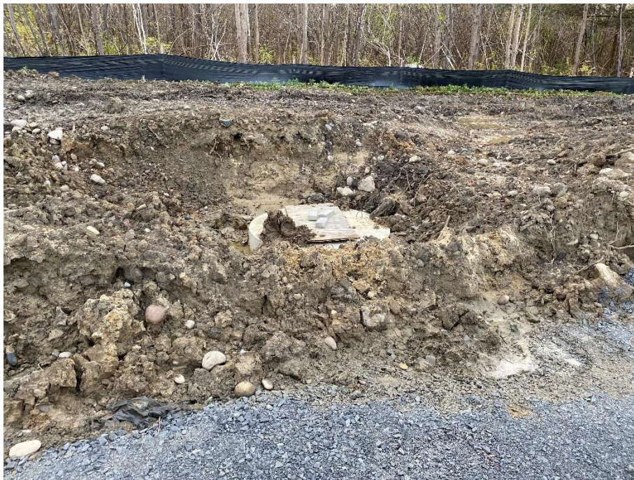
Figure 2 - Add inlet protection around low structures.
