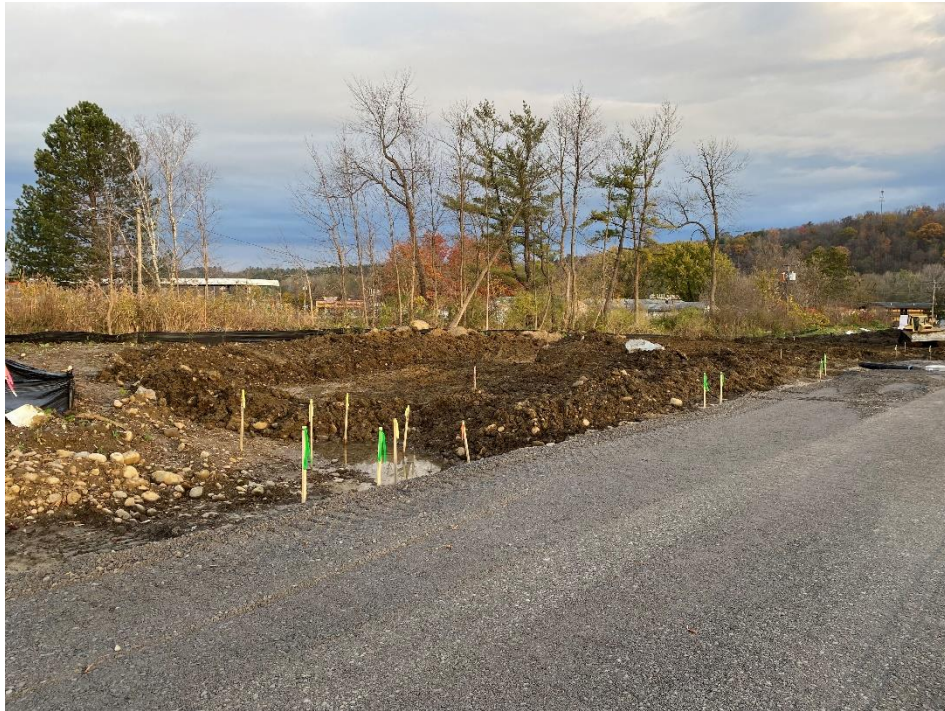
Figure 5 - View of grading for bioretention area along west side of site, looking northwest.
