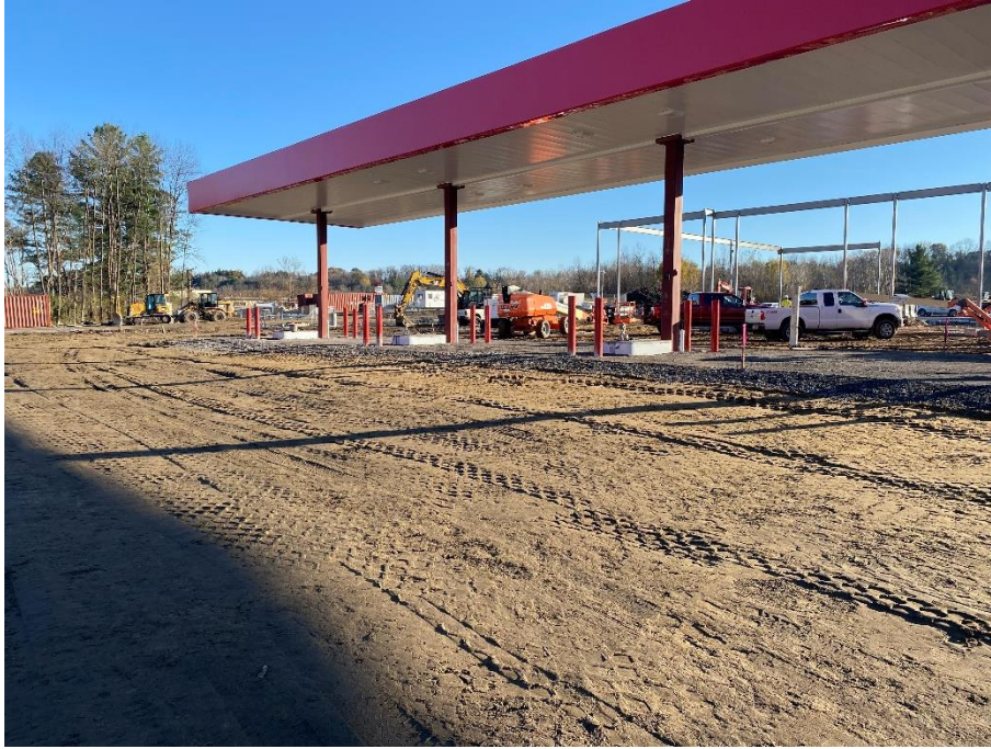
Figure 1 - View subbase grading for gas pump area, looking southeast.
