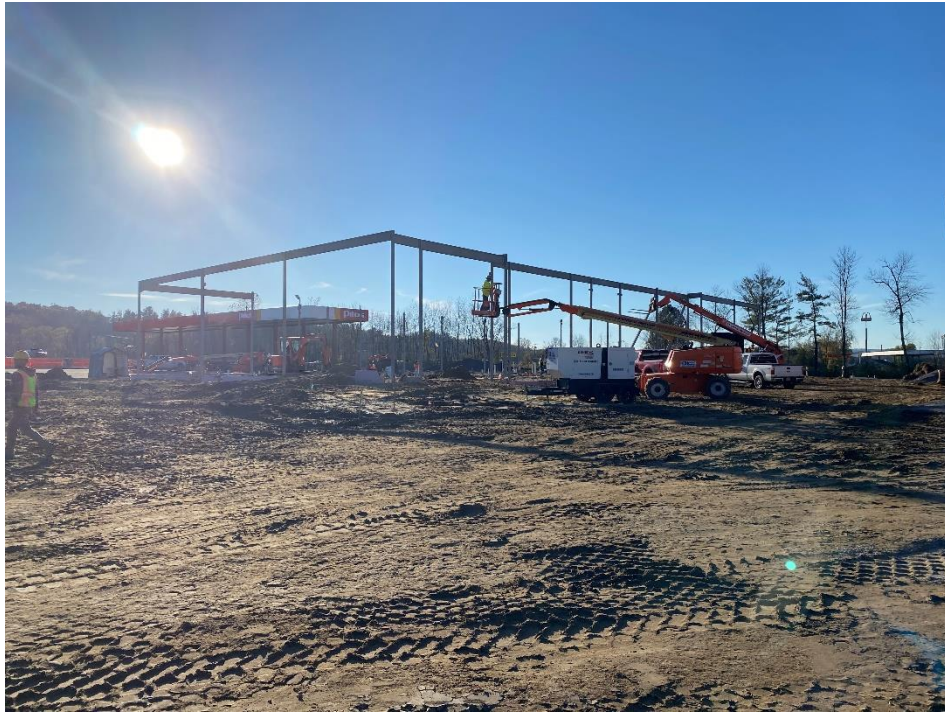
Figure 5 - View of steel erection for building, looking southwest.
