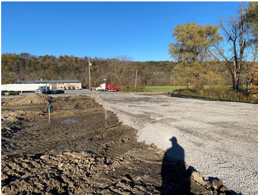
Figure 2 - View of subbase grading for eastern driveway, looking north.
