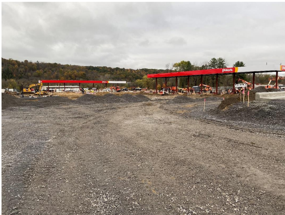
Figure 4 - View of subbase grading along western side of site, looking north.
