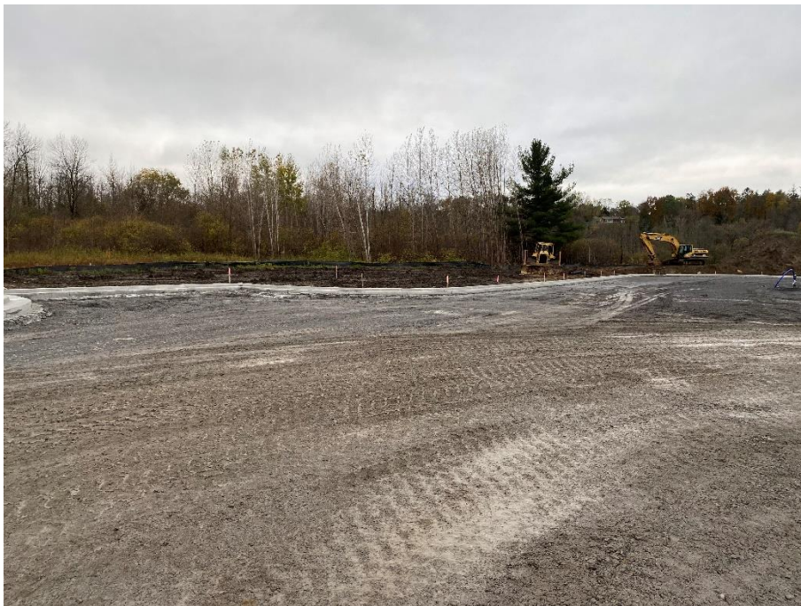
Figure 2 – View of new curb along eastern side of site, looking southeast.
