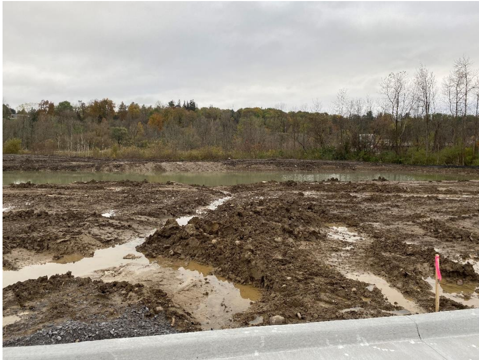
Figure 5 - View of stormwater pond along south end of site, looking south.
