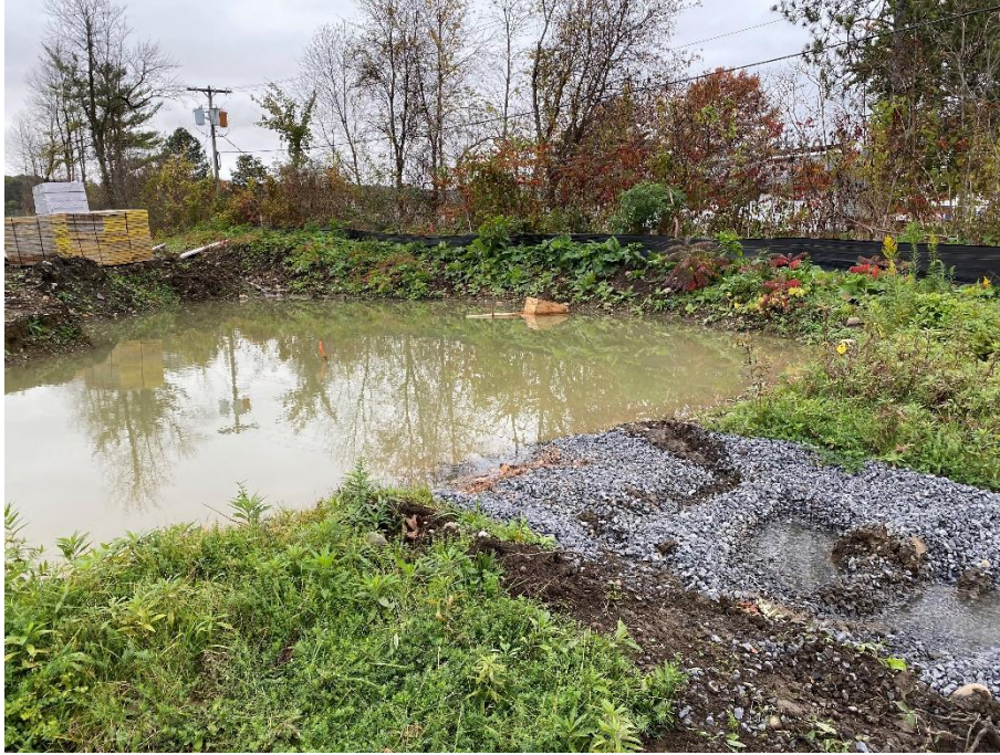
Figure 1 – View of temporary sediment pond in northwest corner of site.
