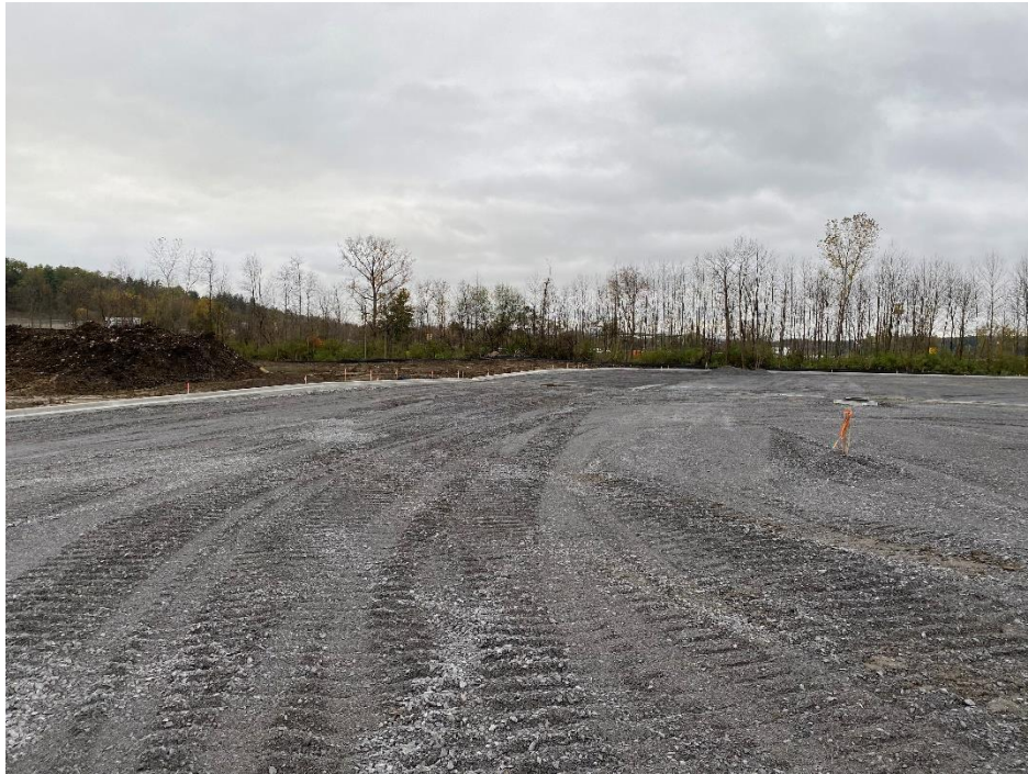
Figure 3 - View of subbase grading and new curb for truck parking area, looking west.
