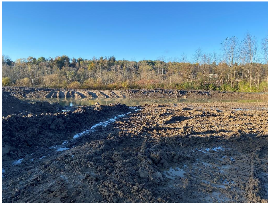
Figure 2 – View of stormwater pond along south end of site, looking south.
