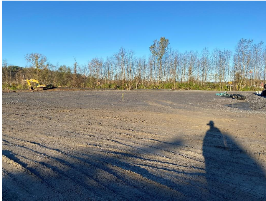
Figure 1 – View of subbase grading for truck parking area, looking west.
