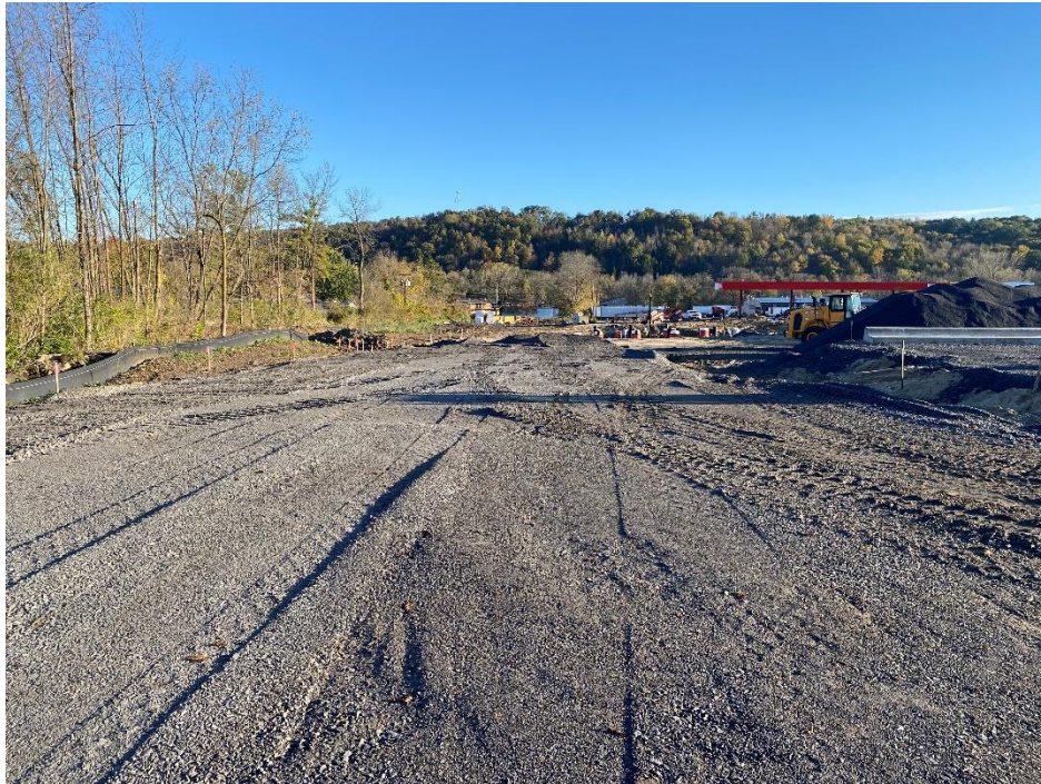
Figure 3 - View of subbase grading for western side of site, looking north.
