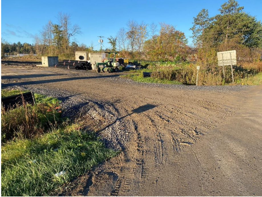
Figure 1 - Refresh the compacted stone for the construction entrance.
