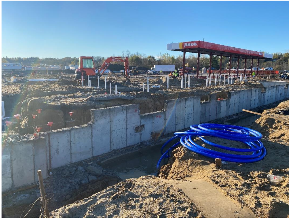
Figure 5 - View of building foundation, looking southeast.
