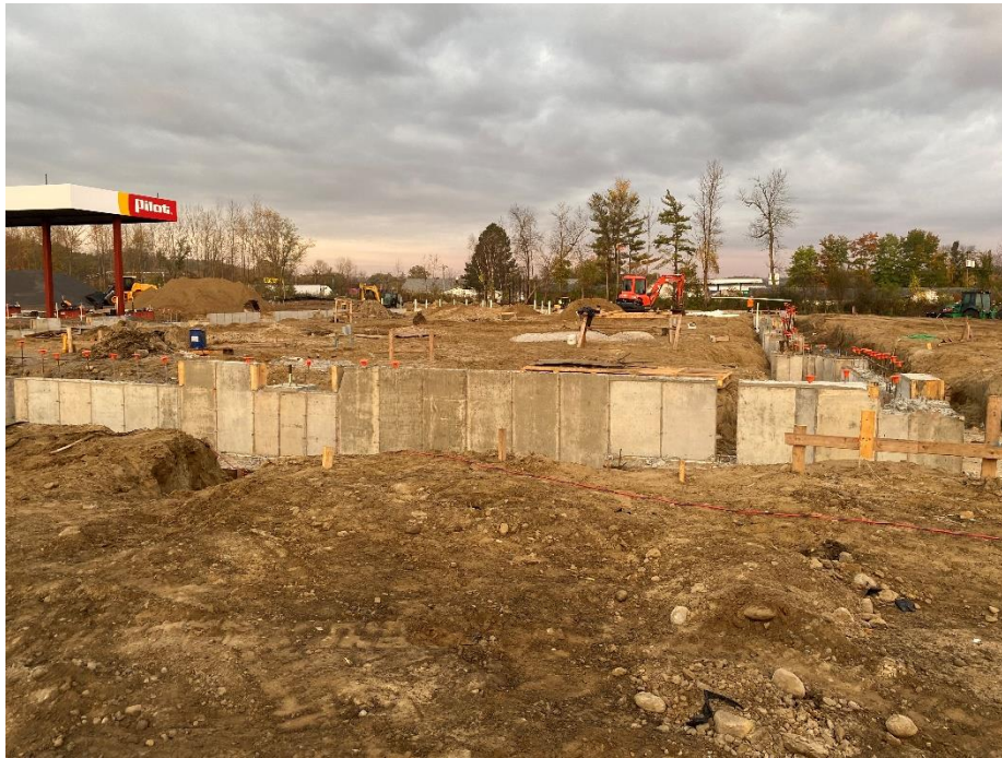
Figure 1 – View of concrete work for building foundation, looking west.
