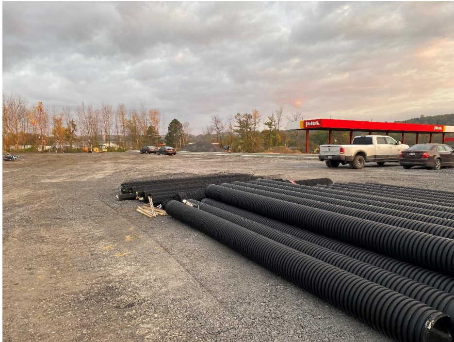
Figure 3 - View subbase grading for back parking area, looking northwest.
