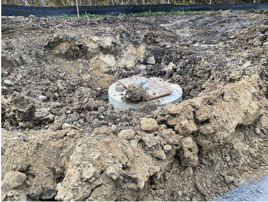
Figure 1 - Add inlet protection around low structures.
