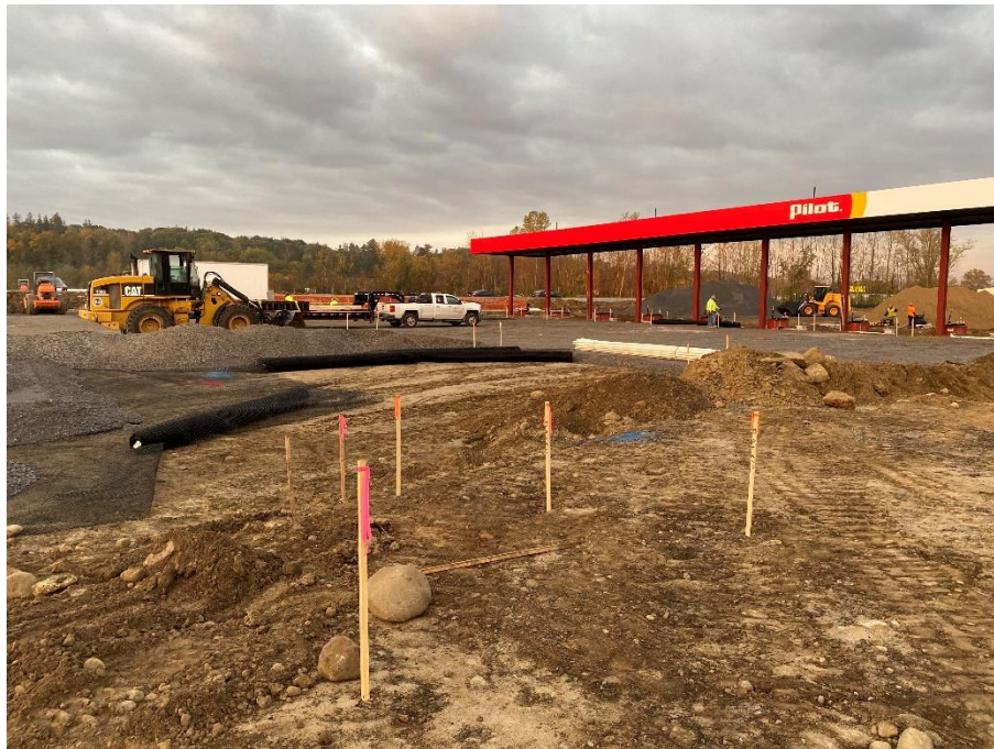
Figure 2 – View of subbase grading for truck fuel pump area, looking southwest.
