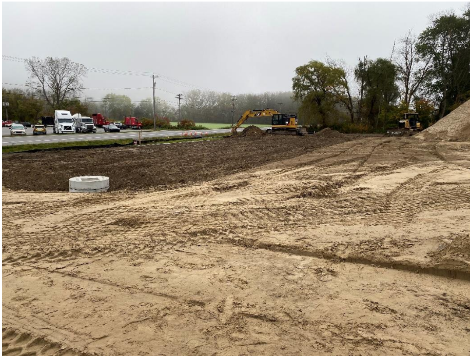
Figure 1 – View of front bioretention area, looking east.
