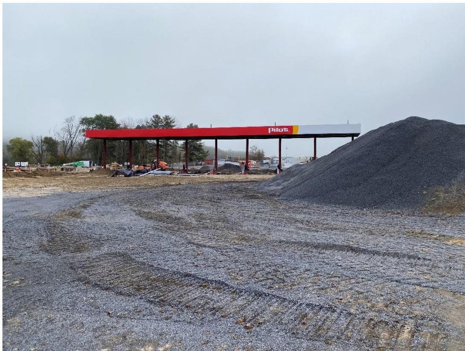
Figure 4 – View of truck fuel pump area, looking east.
