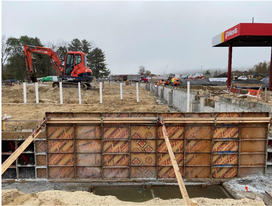
Figure 5 - View of concrete work for building foundation, looking east.
