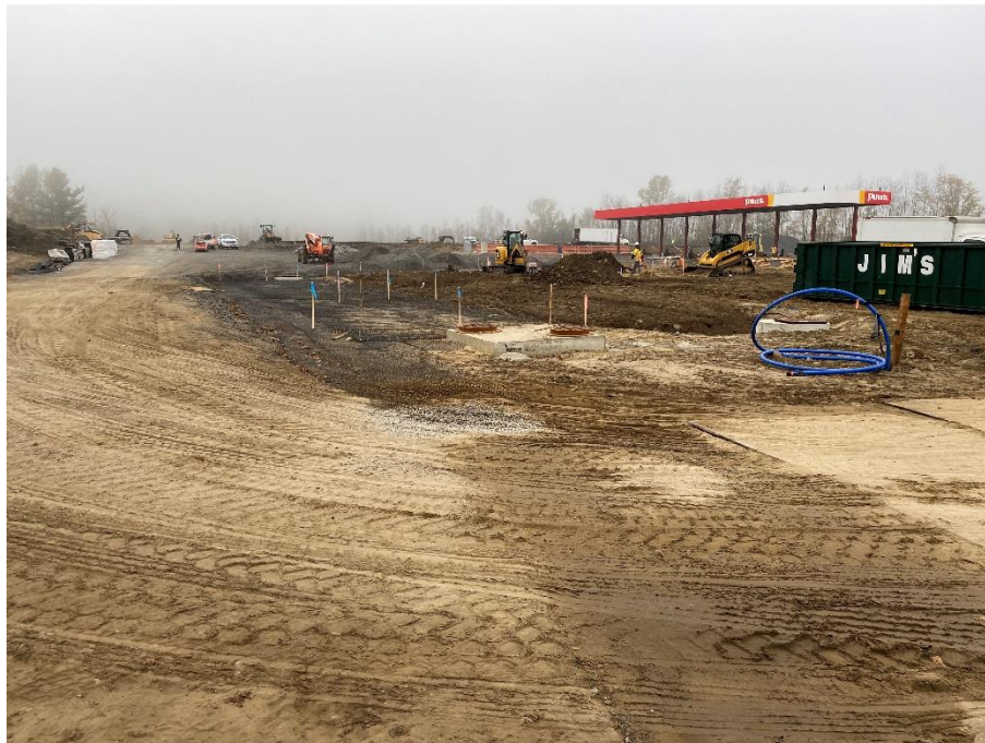
Figure 2 – View of grading for east driveway and stormwater practice, looking south.
