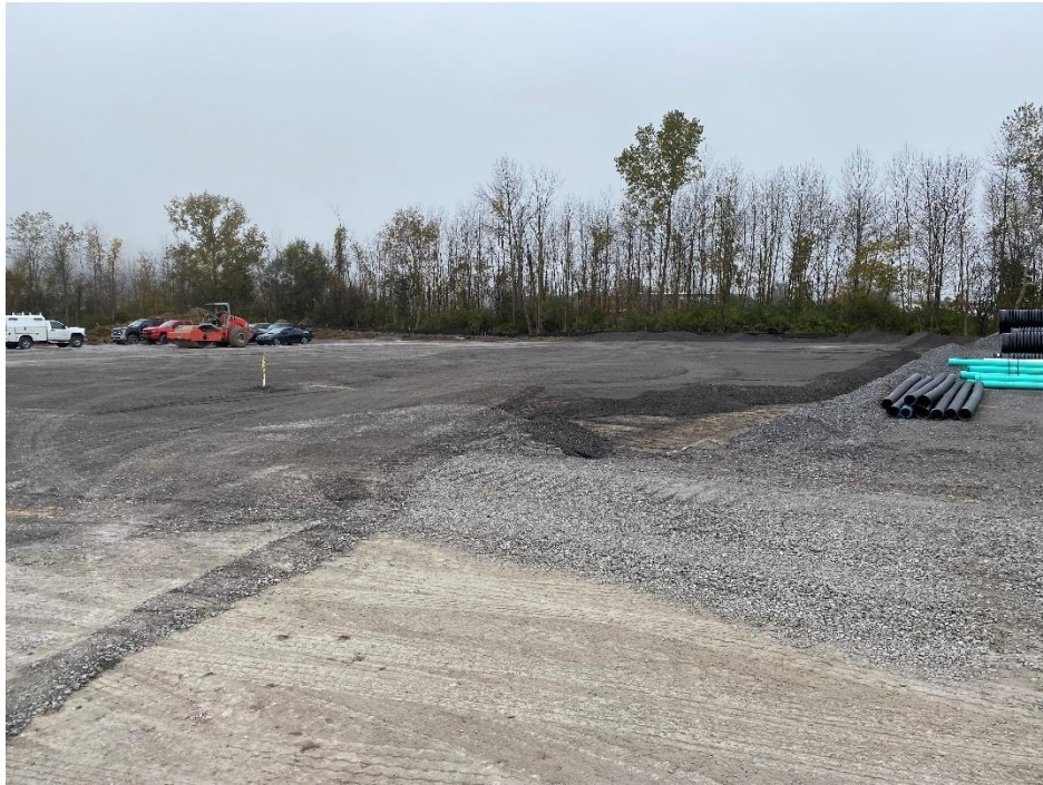
Figure 3 – View of subbase grading for truck parking area, looking west.
