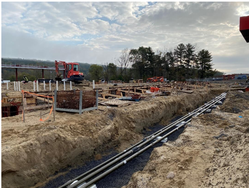
Figure 4 – View of concrete work for building foundation, looking northeast.
