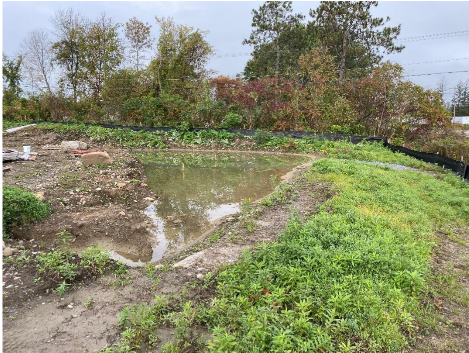
Figure 5 - View of temporary sediment pond in NW corner of site.
