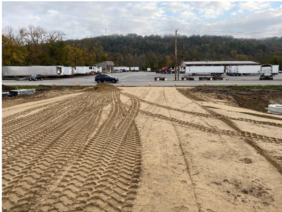
Figure 2 – View of grading for west driveway, looking north.
