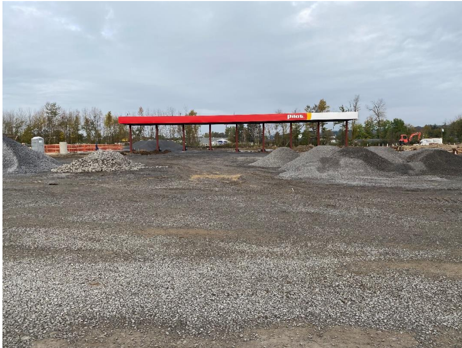
Figure 3 – View of truck fuel pump area subbase grading, looking west.
