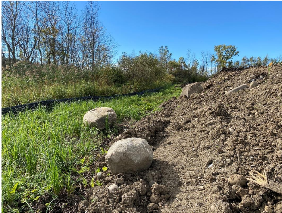
Figure 3 – View of silt fence along south end of site, looking west.
