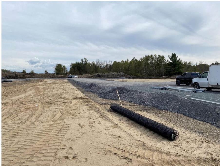
Figure 2 - View of subbase grading for back truck parking area, looking east.
