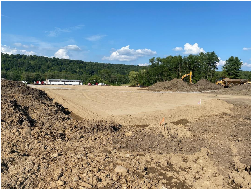
Figure 5 – View of proposed gas pump area, looking north.
