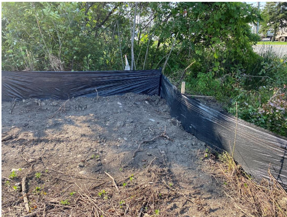
Figure 4 – Repaired silt fence in NW corner of site.
