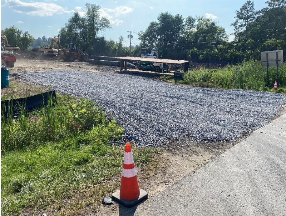
Figure 1 – View of construction entrance at north end of site.
