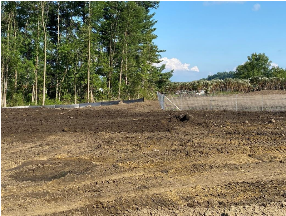
Figure 2 - Continue silt fence along downhill side of laydown area.
