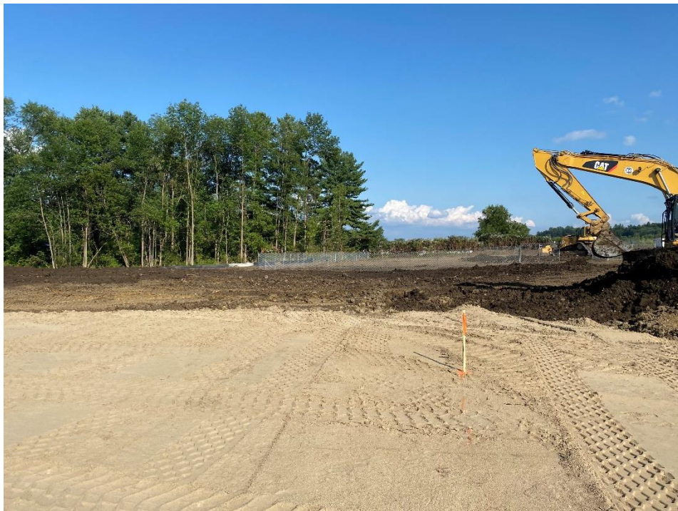
Figure 6 – View of fenced in laydown area, looking east.
