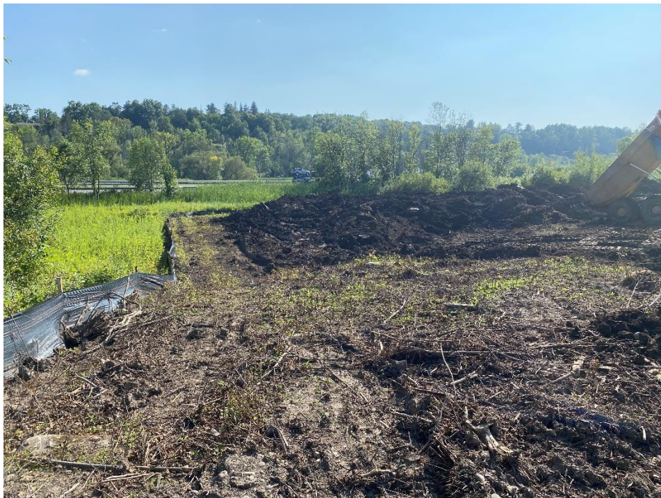
Figure 6 – View of stockpile area at southern end of site.
