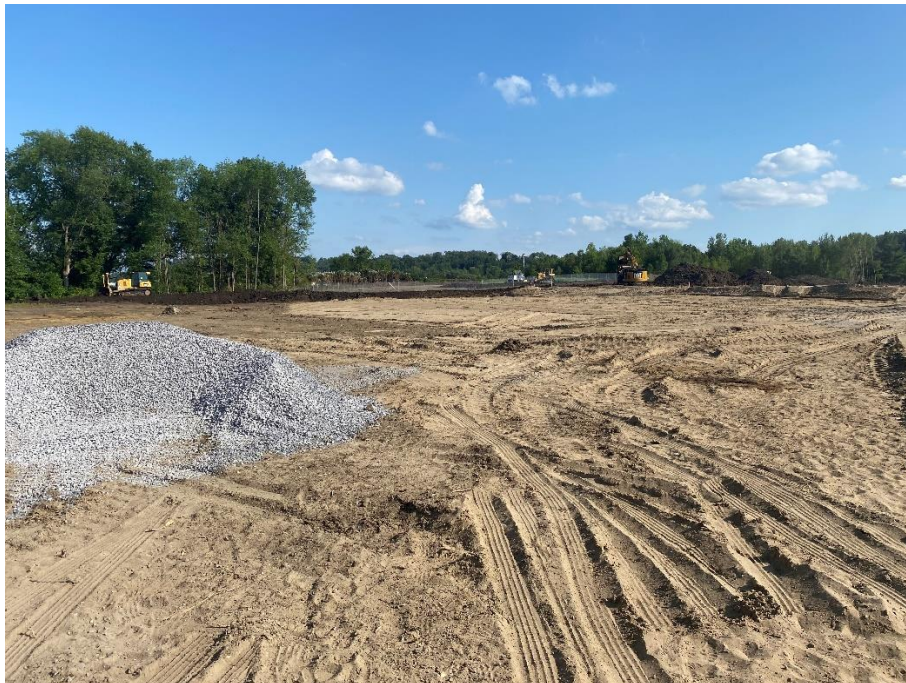
Figure 2 – View of front parking area and laydown area, looking southeast.
