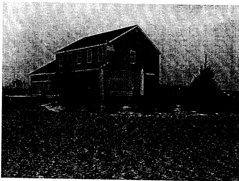
Mohawk Hills residential subdivision on Route 5S
